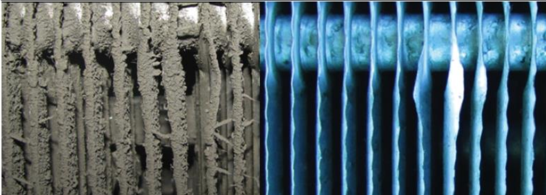
Coils Before Steril-Aire UVC
